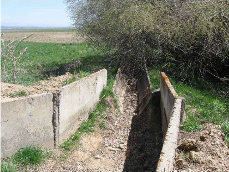
Picture 2. Flume which is subject to rehabilitation, 02 May, 2015
