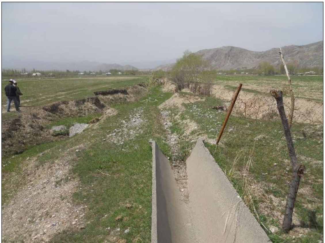
Picture 4. Canal “R-3”, 9 September, 2015
