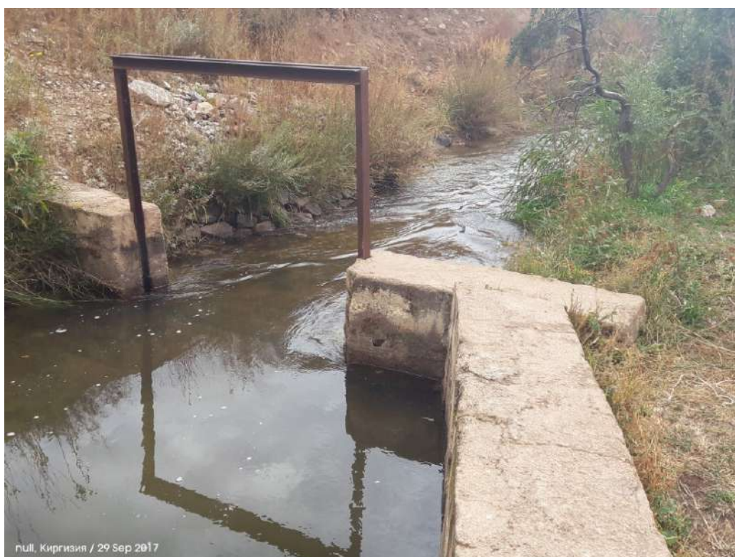
Picture 2. The headwork on canal «Karagul», 29 September, 2017
